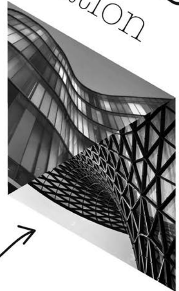
Solar Light Connector, Shangai
